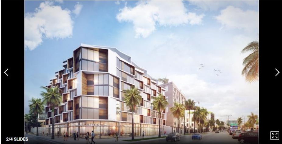
The 153-key AC Marriott Hotel is under construction in Miami's Midtown neighborhood and is set to open in mid-2019. Services and amenities will include restaurant, bar and lounge, business center, meeting space and swimming pool.
