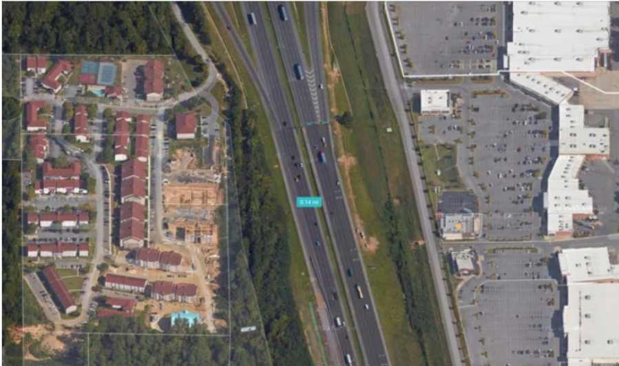
The Colonial Promenade on the right in Fultondale has a new owner after investors cut a $23 million deal.
